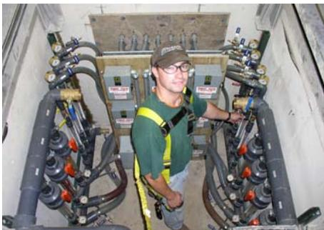
To date, this in-well vapor stripping system is removing approximately 28 pounds of VOCs per day compared to nearby groundwater extraction well removal rates of less than 13 pounds per year. In addition, since the initial startup/shakedown phase, the system has been on-line without interruption except for routine maintenance.
